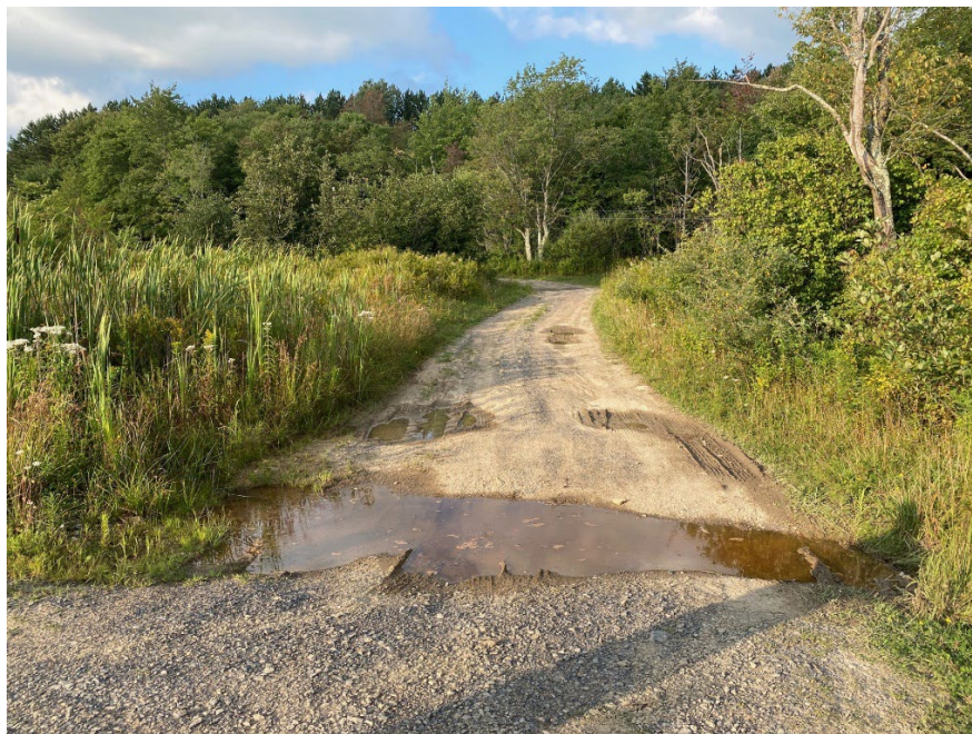
Image 11 - Existing Conditions on WWTP Trail
