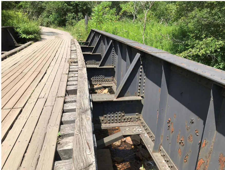
Image 3- Long Run Bridge Existing
