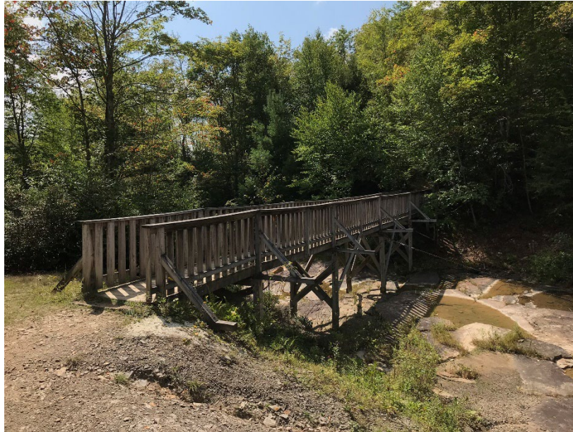
Image 7 - Existing Pendleton Lake Spillway Bridge
